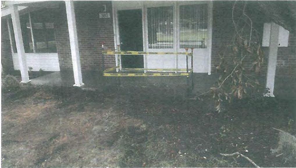
Picture 3: Site after tank removal is completed.
