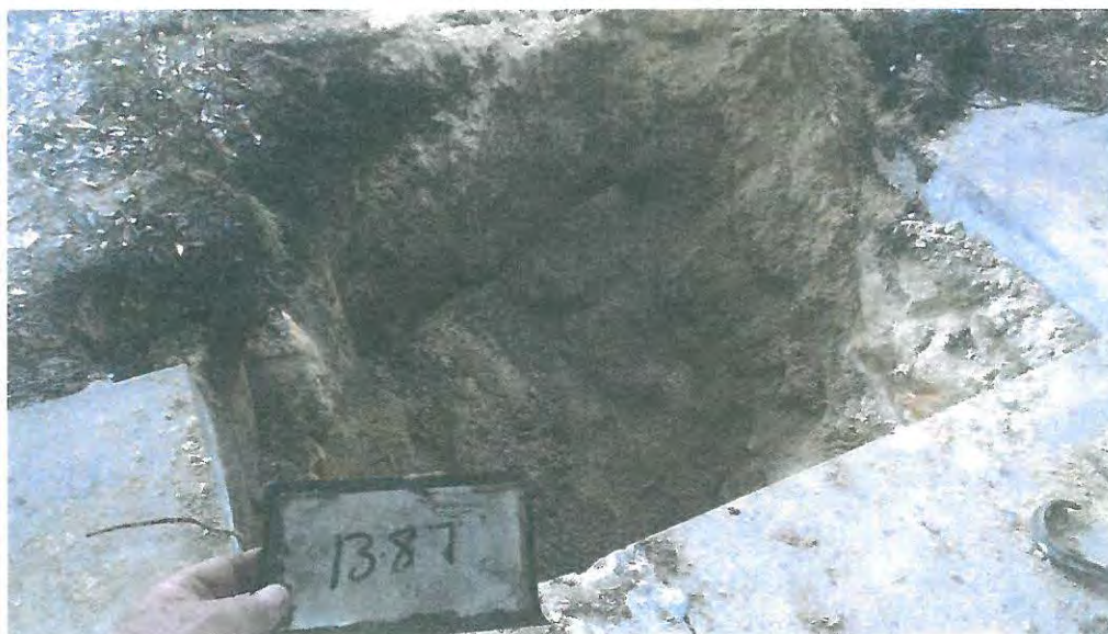
Picture 2: Tank excavation.
